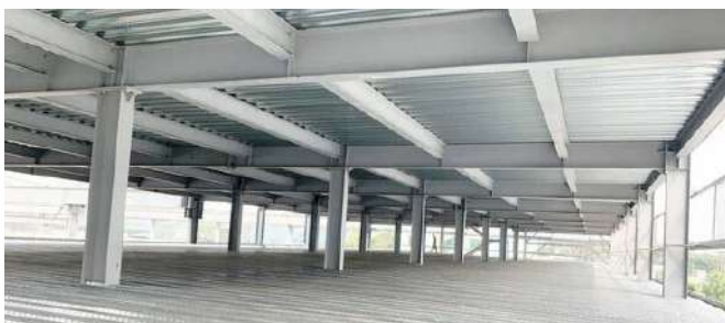
DECK SHEET FLOORING (WITH RCC)
