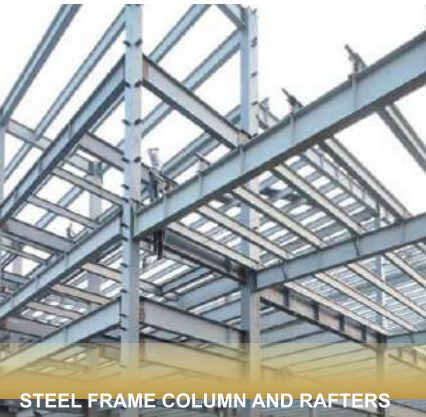
STEEL FRAME COLUMN AND RAFTERS
